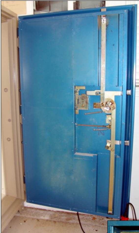
◀ Panel removed. This is a 3-way boltwork, with two door bolts on the opening side, and one each top and bottom.
