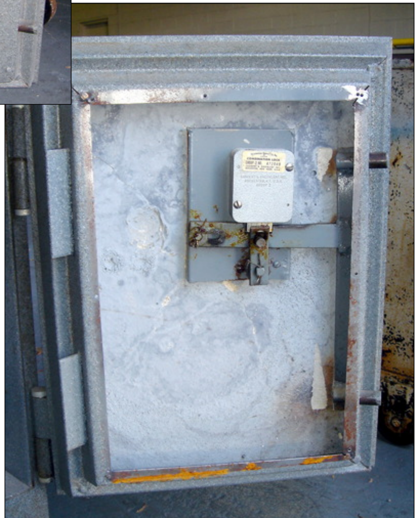
▶ Back panel removed. This is a clean and simple boltwork: two door bolts, both on the opening side, a VD-mounted 6709, and no RL. There is no HP in this door.
