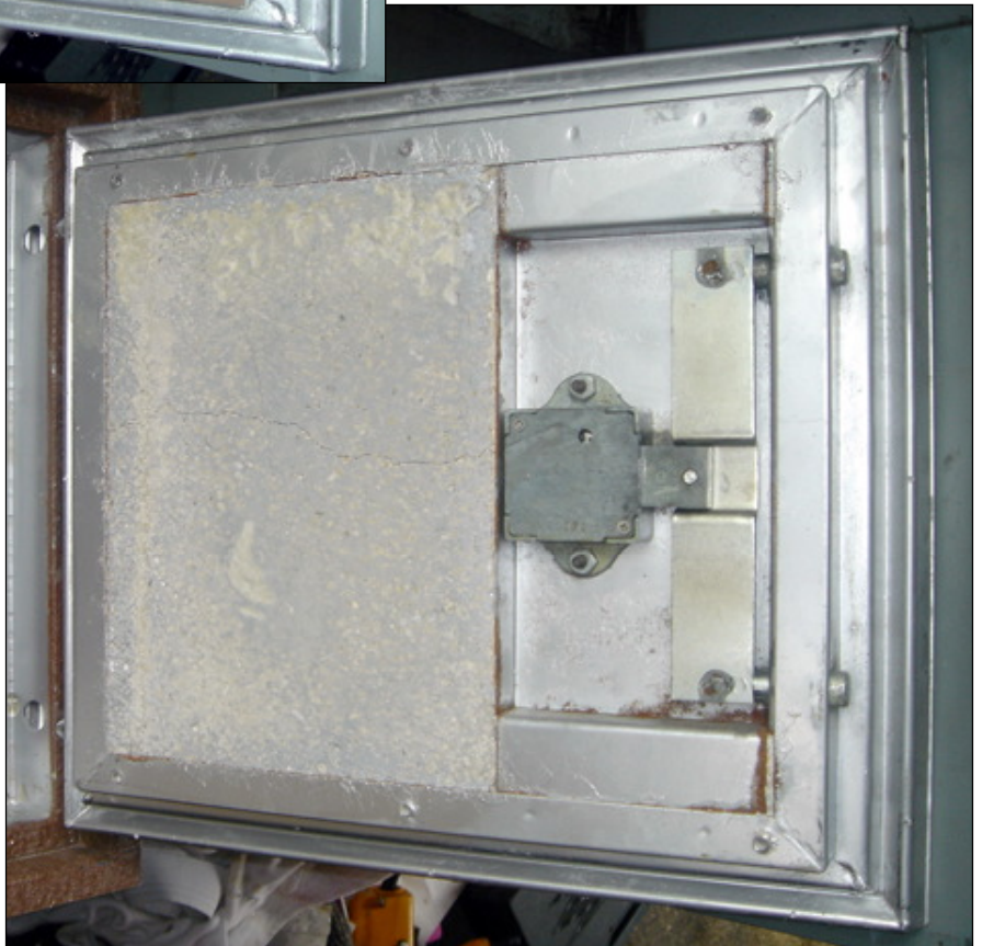
▶ Back panel removed. This is a 1-way boltwork, with two door bolts on the opening side. The lock is mounted RH, and is directly attached to the boltwork.
