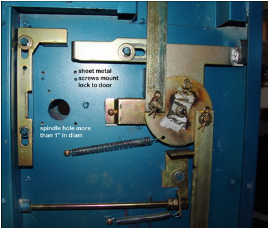
◀ Original lock has been removed.
